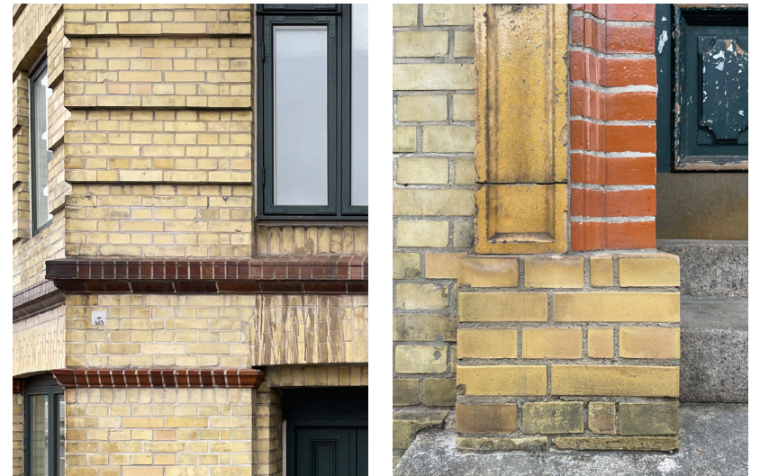
fig. 19 details from the facade of ågade 106, copenhagen
