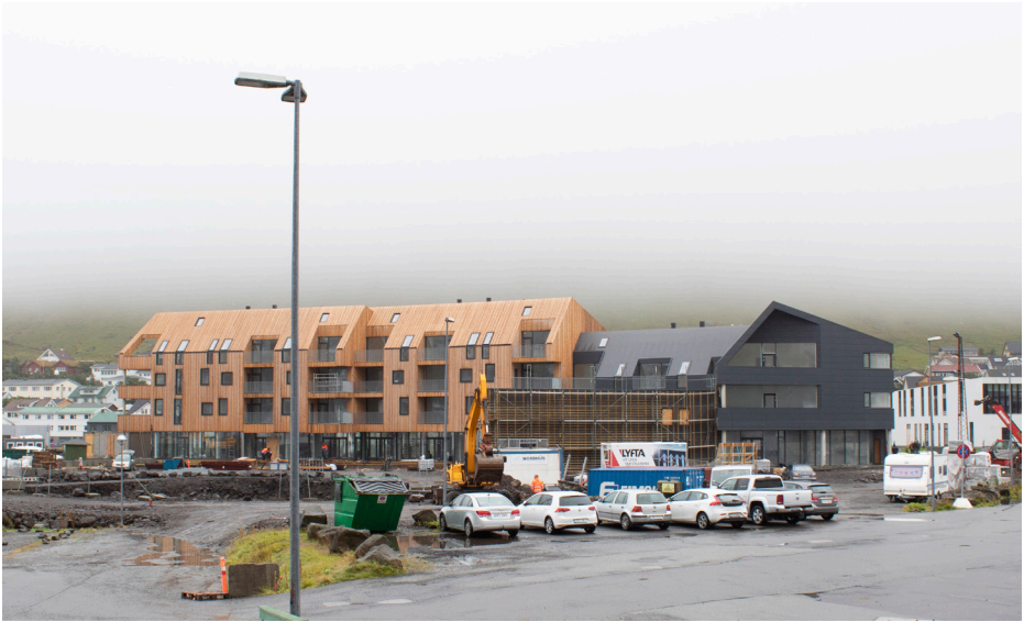
The apartments in Klaksvík under construction
