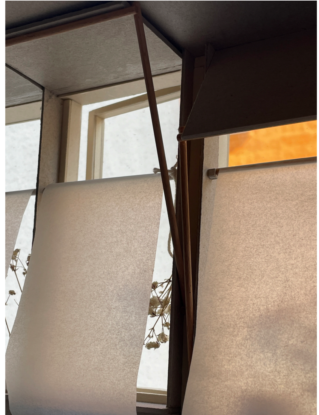
Fig.5.17, upper part of the window- reflect sunlight to the area where occupants need light
