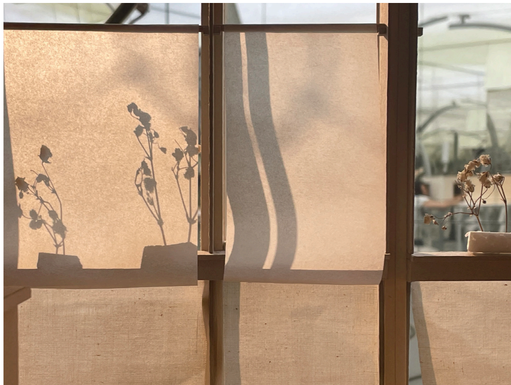
Fig.5.14, middle part of the window- windowsill with two functions of placing objects and curtain box to store the roller blinds
