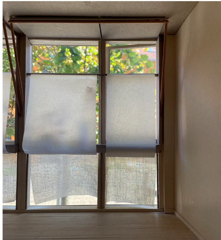
Fig.5.12, middle part of the window-windowsill and roller blind to avoid direct sunlight and gaze from neighboring building
