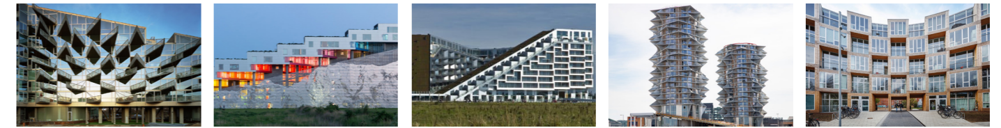
Fig.3.9, 2005, 230 apartments VM Houses Fig.3.10, 2008, 80 apartments The Mountain Fig.3.11, 2010, 475 apartments 8 House Fig.3.12, 2017, 495 apartments Kaktus Towers Fig.3.13, 2018, 66 apartments Dortheavej Residence
