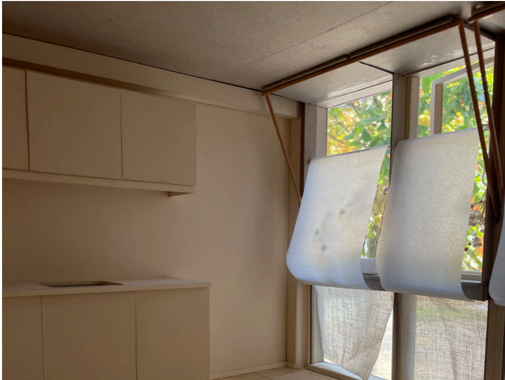
Fig.5.16, below part of the window- avoid the street-level gaze and heat from outside with the curtain drawn from the side
