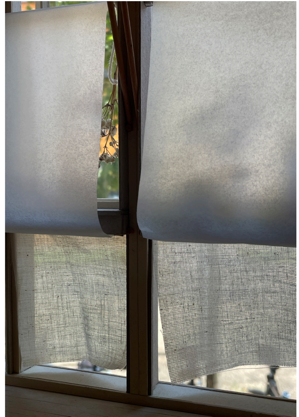
Fig.5.13, below part of the window- avoid the street-level gaze and heat from outside with the curtain drawn from the side
