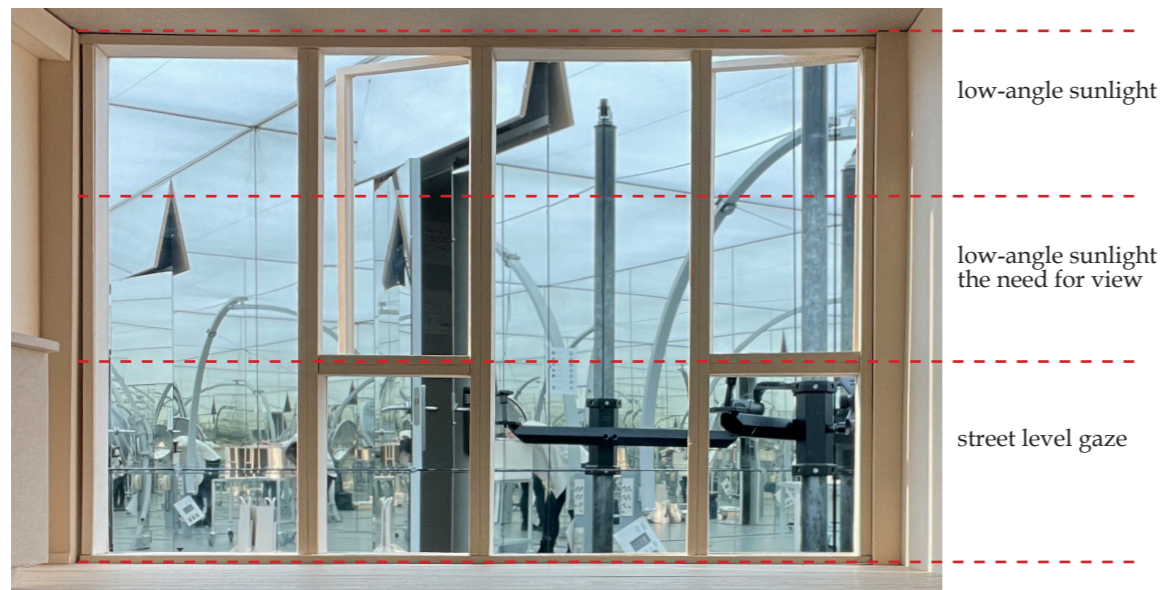
Fig.5.5, division of window according to different need of use
