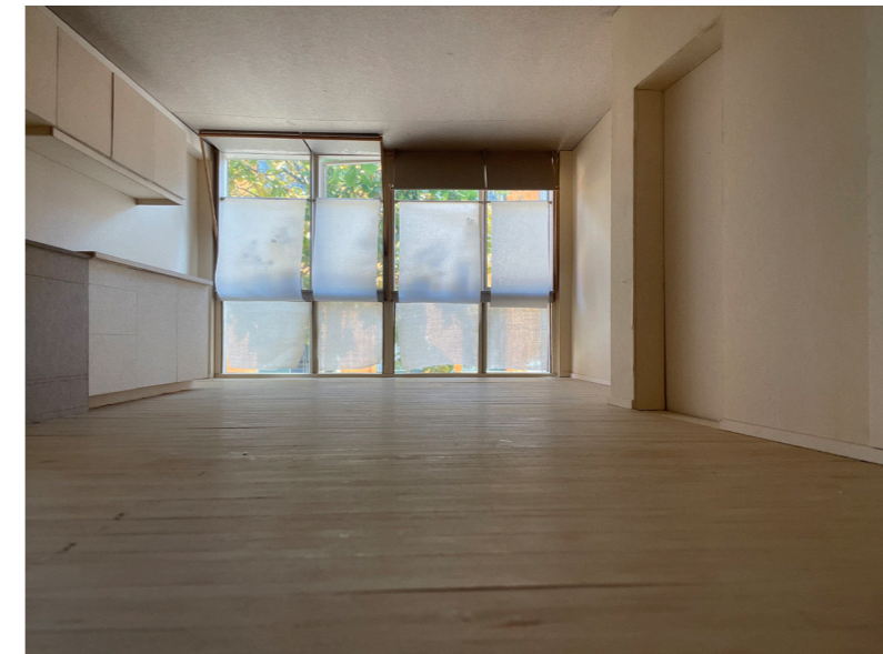
Fig.5.11, flexible adjustment in window settings, the upper part is divided into two components that it can be adjusted base on the direction of sunlight
