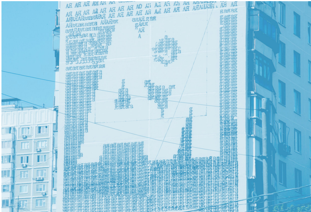
Figure 29. A facade art on of the building in Belyayevo microrayon is a result of a public-private partnership with local artists. The art is a tribute to a local writer Dimitry Prigov representing one of his Poetrygramms.
