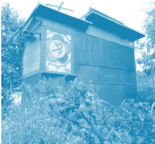
Figure 26. A dovecote in one of the Yasenevo courtyards before demolition.
